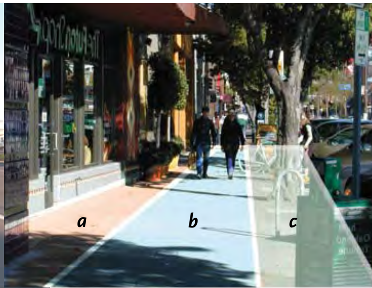
SIDEWALK DESIGN—SHATTUCK AVENUE, BERKELEY, CALIFORNIA a) frontage zone: canopy & merchandise display; b) through pedestrian zone; c) furnishings zone
